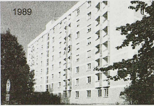
Fig. 6. Western façade of object 16 (old people's home in Munich) in September 1989, three years after application of an ETICS and another 15 years later in November 2004 (the difference in colour does not mean that the façade has been repainted, it is due to coloration problems with digital photography). The formation of algae is clearly visible especially in areas intensely exposed to rain (see arrow and Fig. 7)
