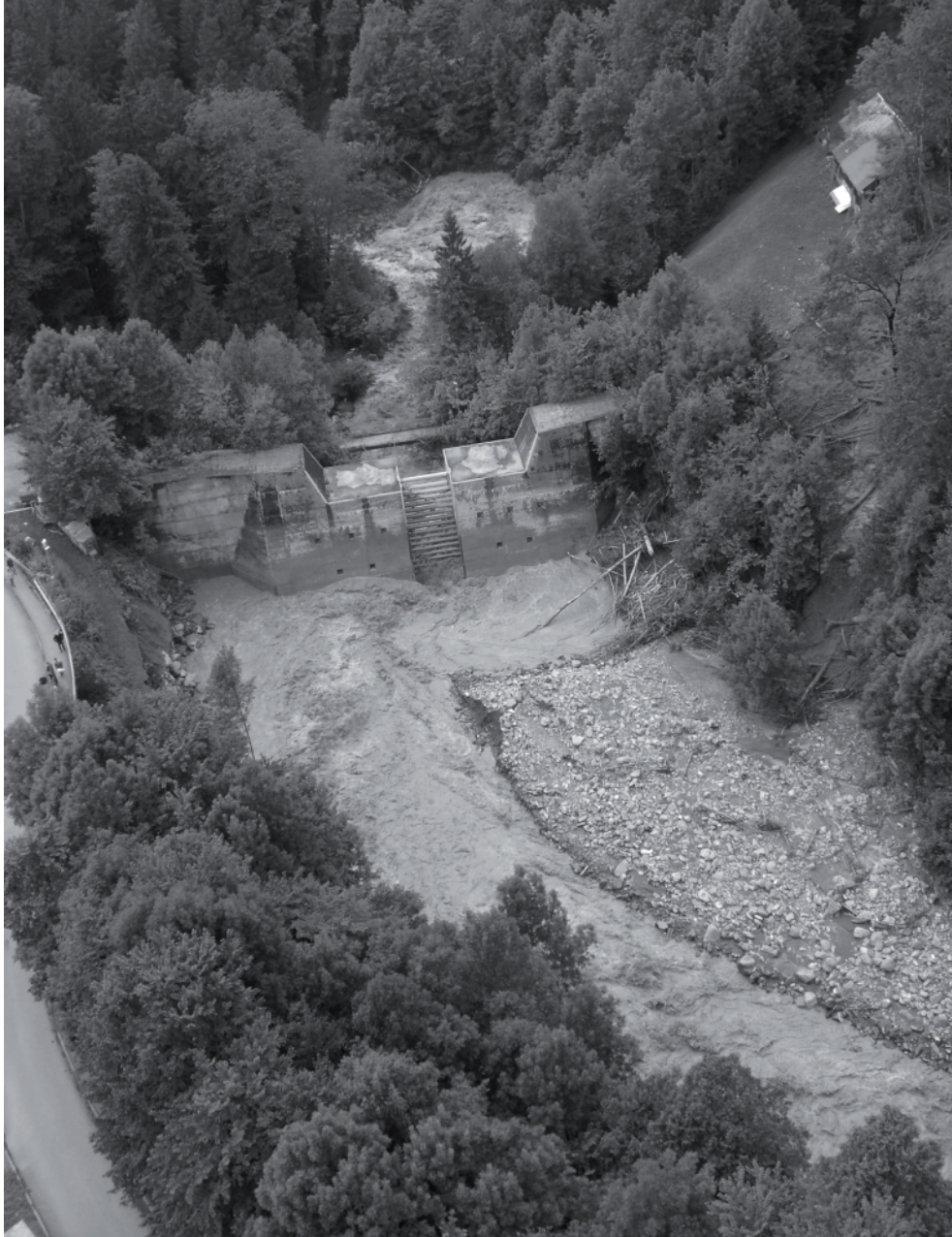
FIGURE 3. Sediment detention basin 'Stiglisbrücke', about 4 km upstream of the confluence, towards the end of the flood. A large part of the deposition visible on the right was flushed later during receding flow (courtesy Canton of Uri)
