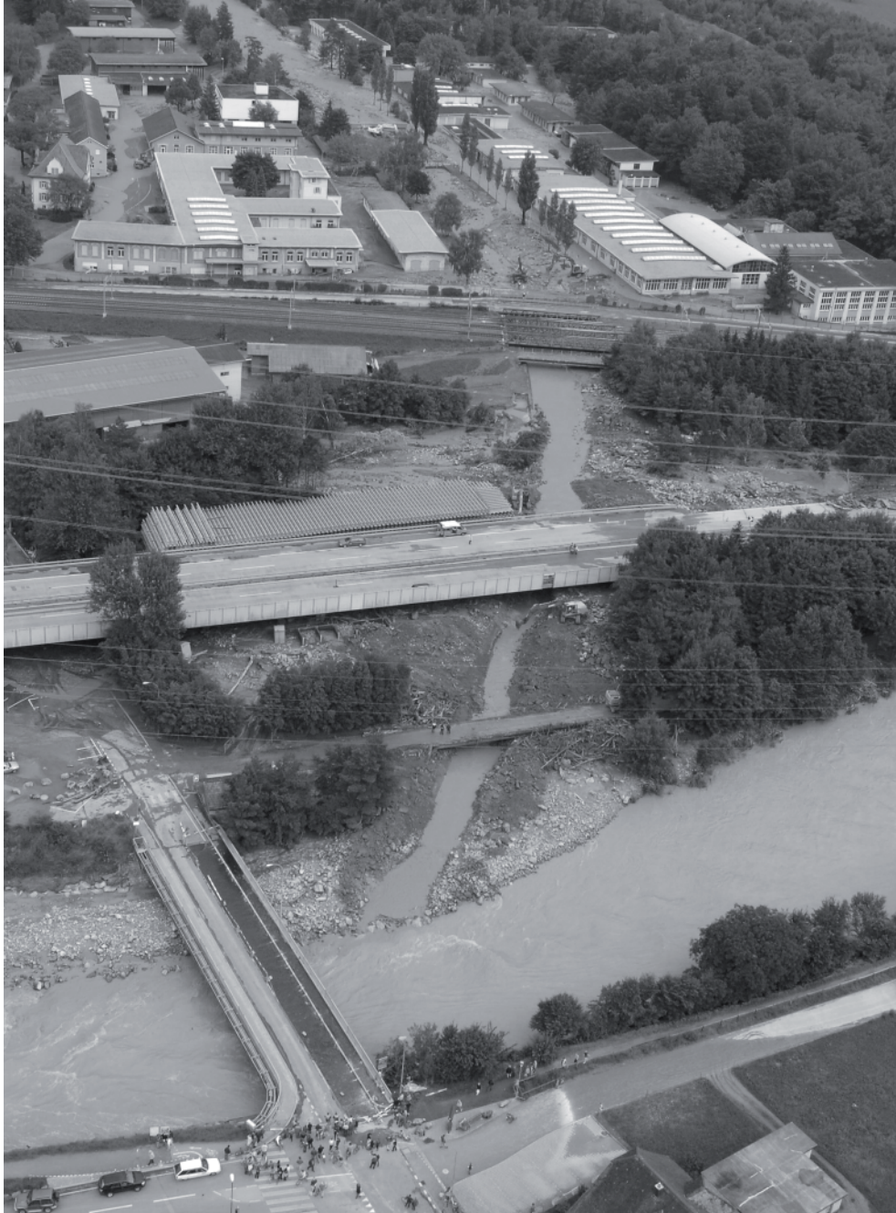
FIGURE 1. Confluence of the Reuss and Schächen rivers after the flood of August 22/23, 2005. The lined masonry channel of the tributary is completely filled with sediment, what caused inundation of the industrial zone in the background (courtesy Canton of Uri)
