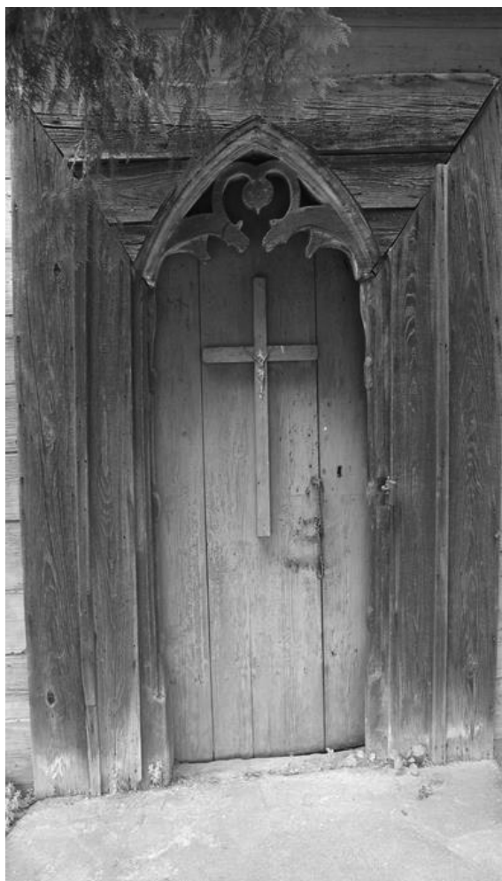
Fig. 3. The Gothic portal ( Quercus sp. ) in chapel in Bialynin transferred from the defunct parish church
