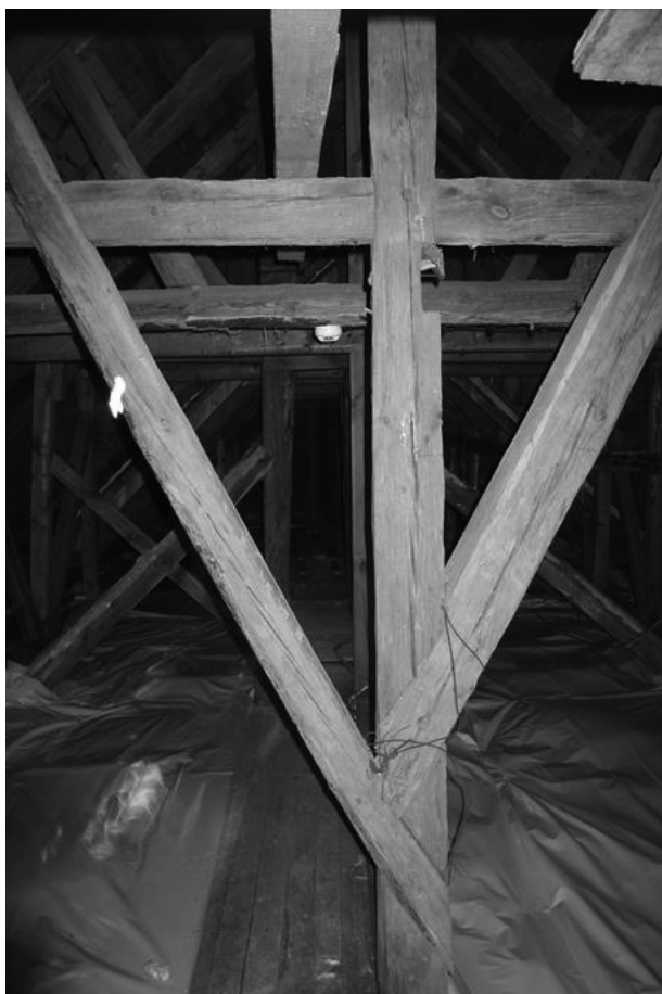
Fig. 2. Part of original roof structure in churches in Rębertów
