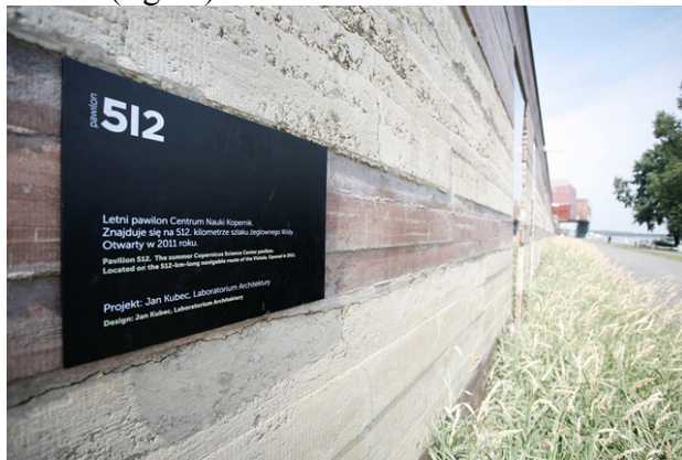
Fig. 1. Wall of Pavilion 512 of Copernicus Science Center in Warsaw, made of clay [www.512.kopernik.org.pl/pawilon-512.html]
