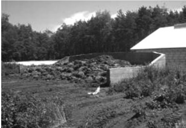
FIGURE 2. The dunghill with inappropriate discharge of leachate into the tank and the lack of adequate protection zone (photo: K. Wiśniewski)
