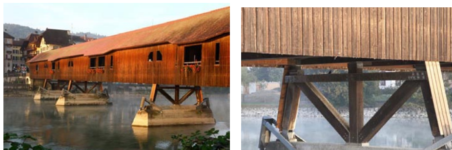
Figure 1. Aare Bridge – general view and support construction
