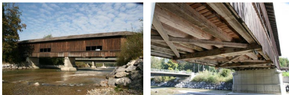
Figure 3. Gohlhaus Bridge – general view and deck construction
