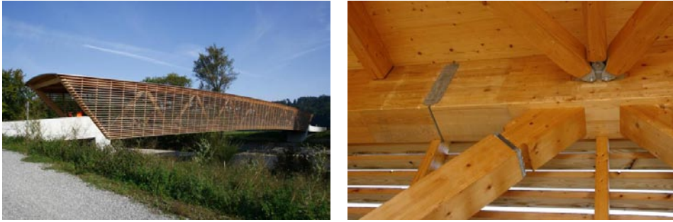
Figure 4. Neumatt Bridge – general view and connection
