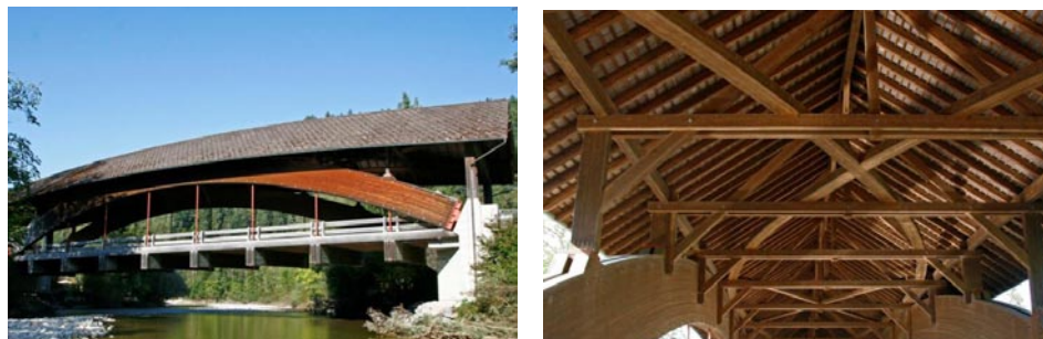
Figure 2. Baubenei Bridge – general view and roof construction
