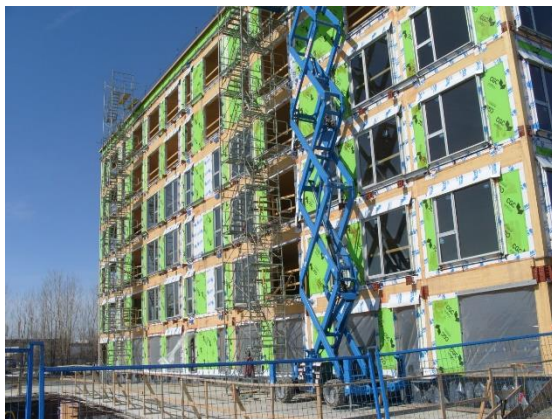
Figure 4. The multi-storey building in Montreal ( Fot. S. Krzosek )
