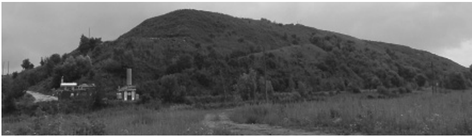
FIGURE 5. The effect of the hydroseeding method applied on Radiowo landfill
