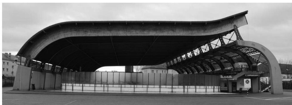
Figure 1. View of the roof of the public ice skating rink
