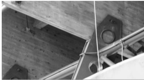
Figure 4. Displacement of the central girders on the top support
