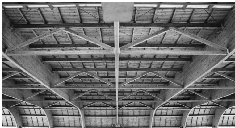
Figure 2. View of the roof stiffenings
