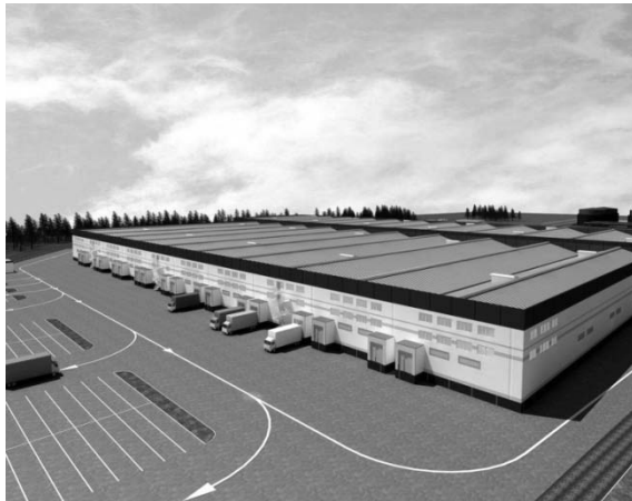
Fig. 5. Logistics terminal building
