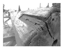
Fig. 2. Damage to monument due to the fastening system
