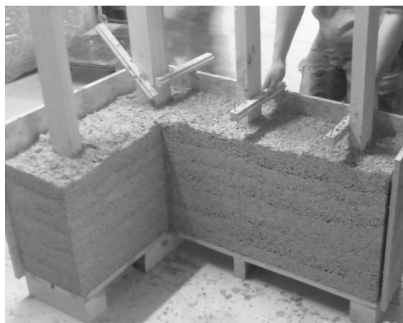
Figure 7. The mixture of lime-hemp composite placed in the wall shuttering
