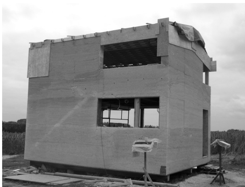
Figure 10. Erecting the first house in Poland completely insulated with hemp
