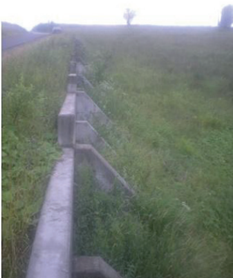
FIGURE 7. Retaining wall on the landslide Milówka Nielewida (Dziedzic and Golan 2016): a – upper retaining wall; b – middle retaining wall with an absorption well
