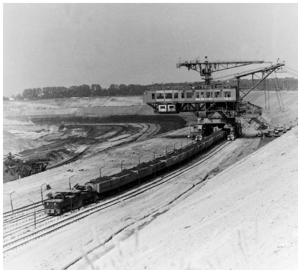
FIGURE 3. Traction mode while excavating in mine “Cospuden” (1985)
