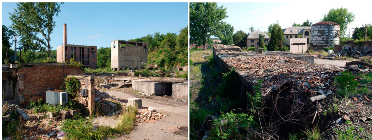
Fig. 3. Left: Transformer station (in front), the boiler-house and the coal-pillbox (background); right: demolished coal-press (in front) and the bitumen tank.
