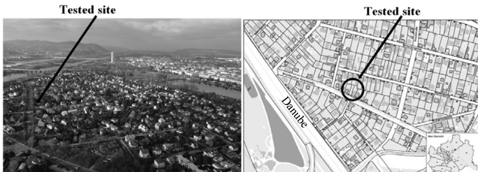
FIGURE 1. View of the Bruckhaufen housing estate and a spatial development plan of the area (source: Chagià José – Vienna, commons.wikimedia.org; Stadt Wien – ViennaGIS)
