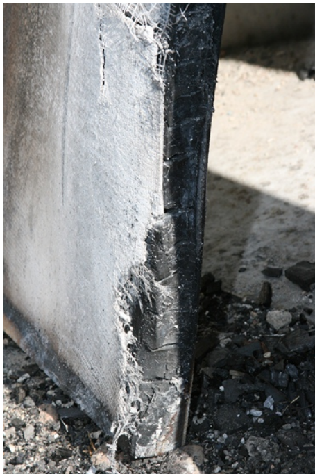
Fig. 3. CWM covered with magnesite panel after the testing
