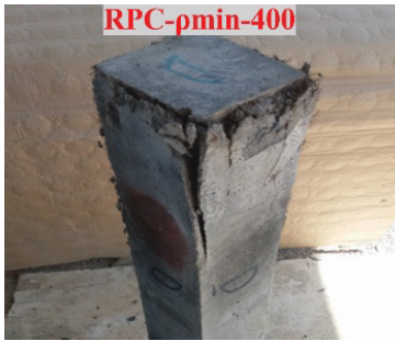
FIGURE 6. Typical crack pattern of pure axial concentric load columns
