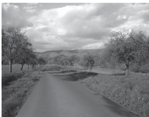
FIGURE 11. Road with small trees that show a tendency to develop ill-formed forks, but are situated a safe distance from the road
