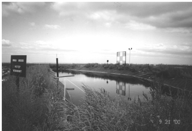
FIGURE 9. The leak-tight basin for leachate recirculation in the landfill surface
