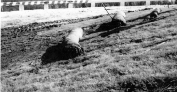
FIGURE 12. Grass carpets introduction into the landfill slopes
