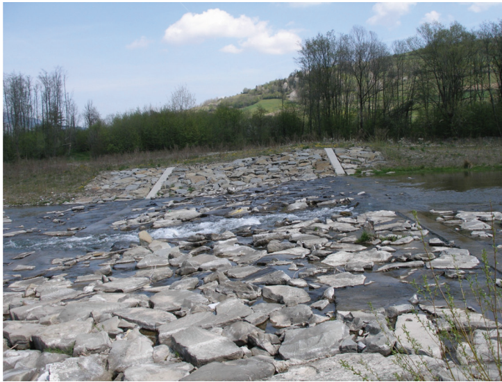
Photo 1. The bloc ramp on Porebianka stream – please notice curtain walls, photo A.Radecki-Pawlik
