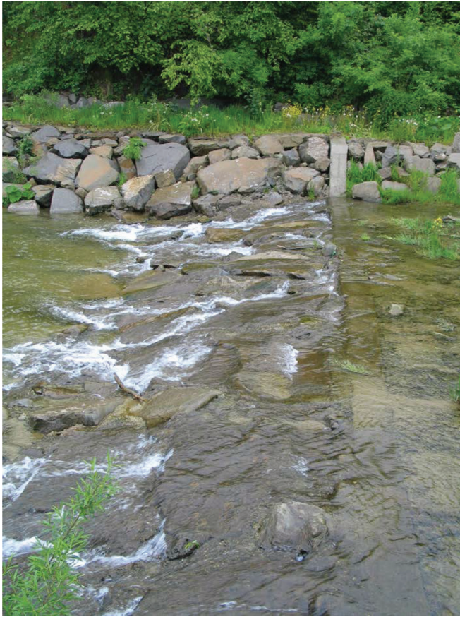
Photo 2. The bloc ramp on Bienkowka stream – please notice upstream edge of a curtain wall, photo A.Radecki-Pawlik
