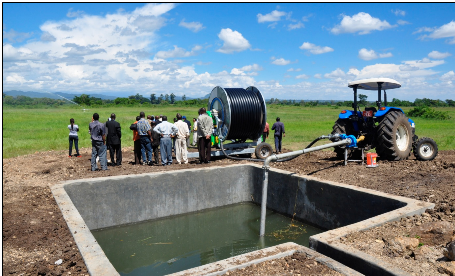
Photo 1. Basic elements of II stage of implemented irrigation project (water reservoir, tractor operated pump and hose reel irrigator)
