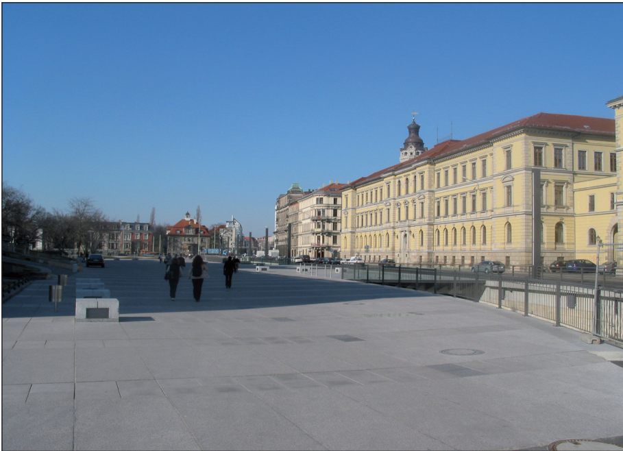
Fig. 1 Soil sealing of a public open space in Leipzig, Germany
