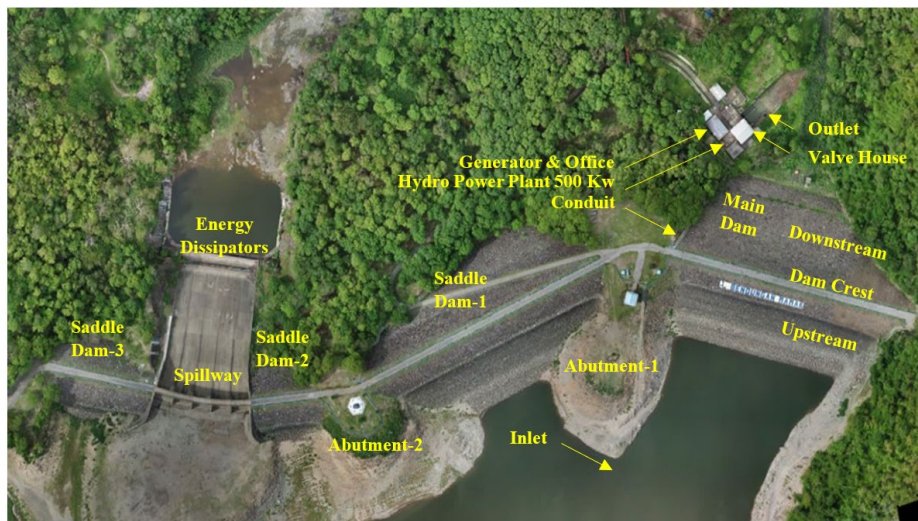
Fig. 2. Bird's view of the Mamak Dam
