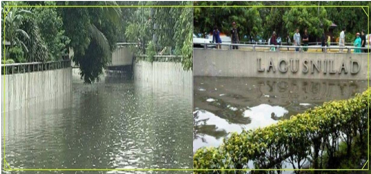
Figure 2. Floods in Lagusnilad's drainage system
