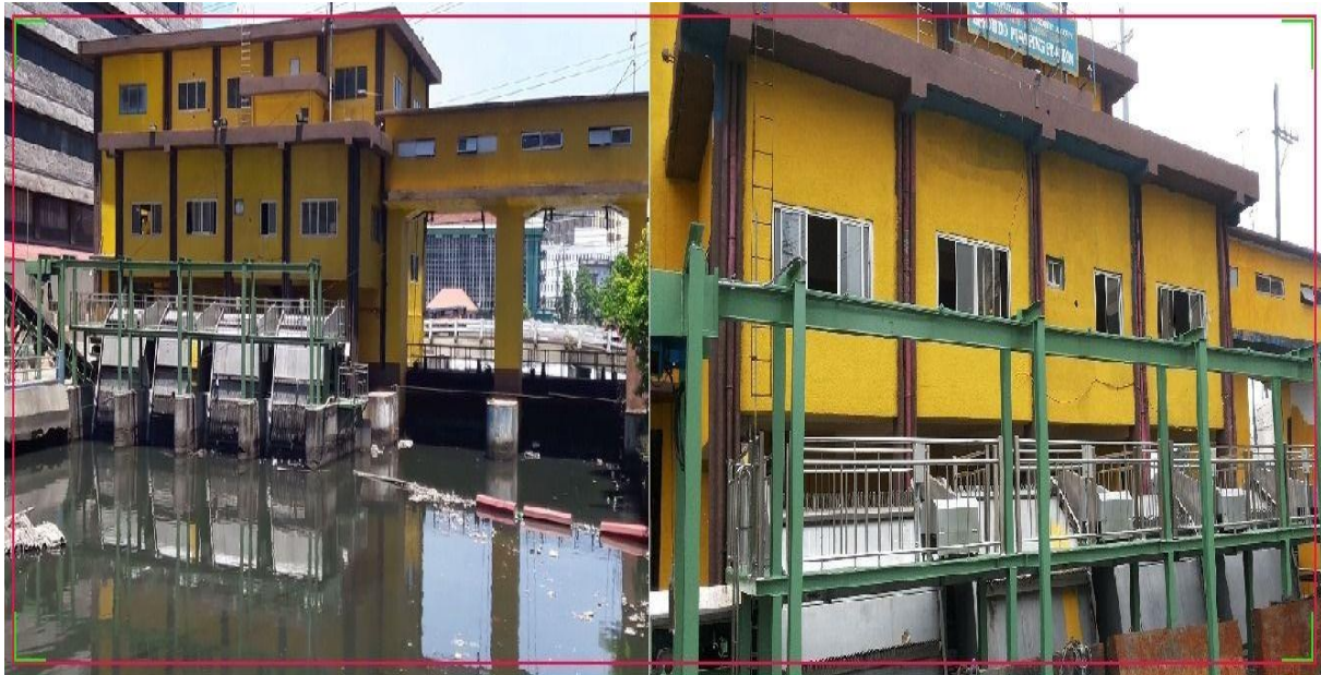
Figure 4. Binondo pumping station
