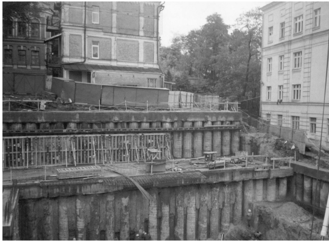
Fig.1. The filler walls fastening for foundation pit at construction site
