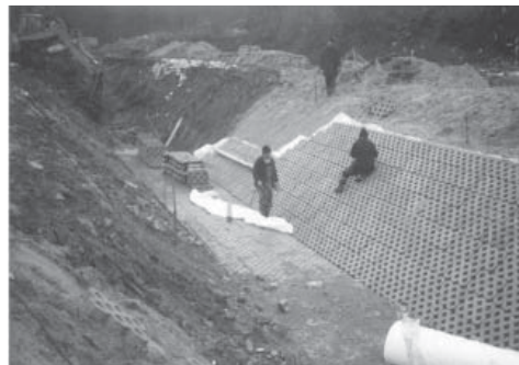
RYSUNEK 2. Umacnianie skarp rowu płytami EKO na geowłókninie i podsypce, 2000 rok FIGURE 2. Ditch's slope reinforcement with concrete slabs on geotextile and mineral sand, 2000
