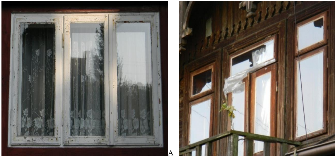
Figure 10. A triple-unit window: single-casement window combined with a double-casement window: A- Poetycka 5 (No.59), and single-unit windows with transom with a more complex central unit: B- Andriollego 66 (No.2)
