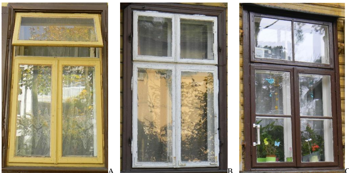
Figure 5. Opens with pivoting upper part: A- Samorządowa 8 (No.66), B- Bagatela 27 (No.3), C- Mickiewicza 25 (No.41)
