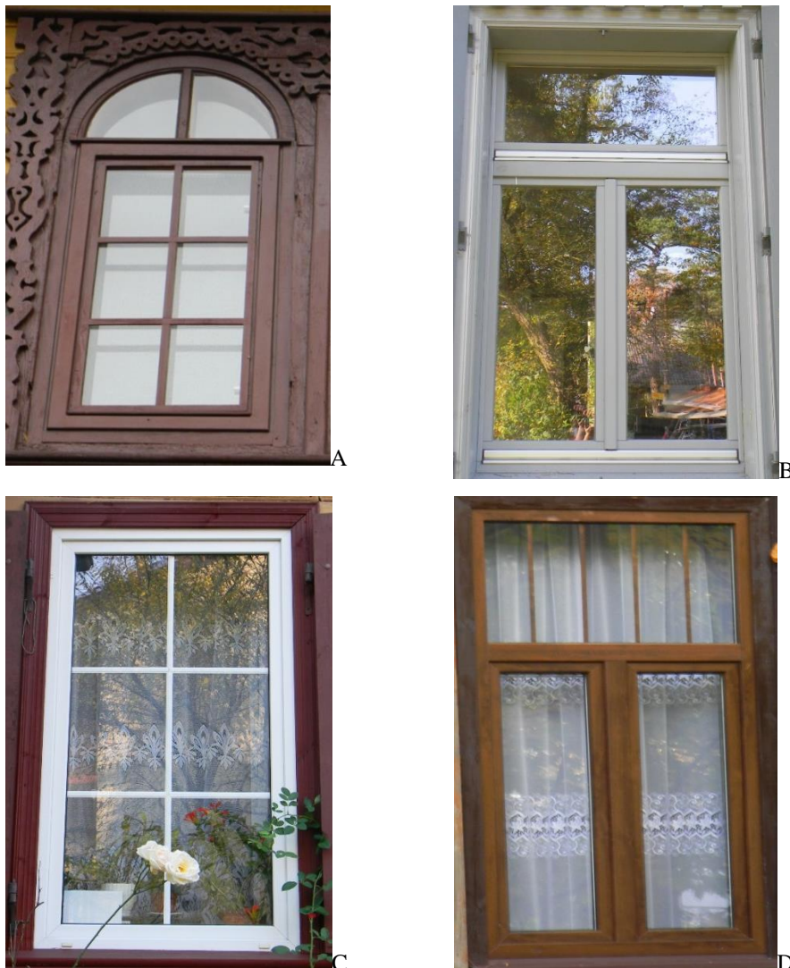
Figure 2. New windows made in traditional style in buildings at: A- Kraszewskiego 101 (No.31), B- Lelewela 7 (No.33), C- Poetycka 5a (No.59) and D- Kościuszki 7 (No.24)
