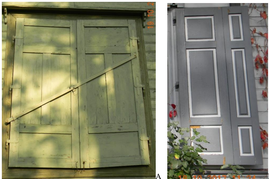
Figure 18. Shutters with single, wide shutters on each side: A- Mała 3 (No.38), and shutters divided into with two asymmetrical casements on each side, connected with hinges: B- Lelewela 7 (No.33).
