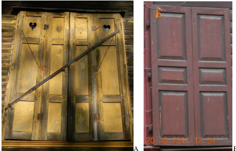
Figure 19. Shutters made of two casements each, connected with hinges: A- casements of similar width, Jaremy 5 (No.14) and B- of identical width, Mickiewicza 35 (No.44)
