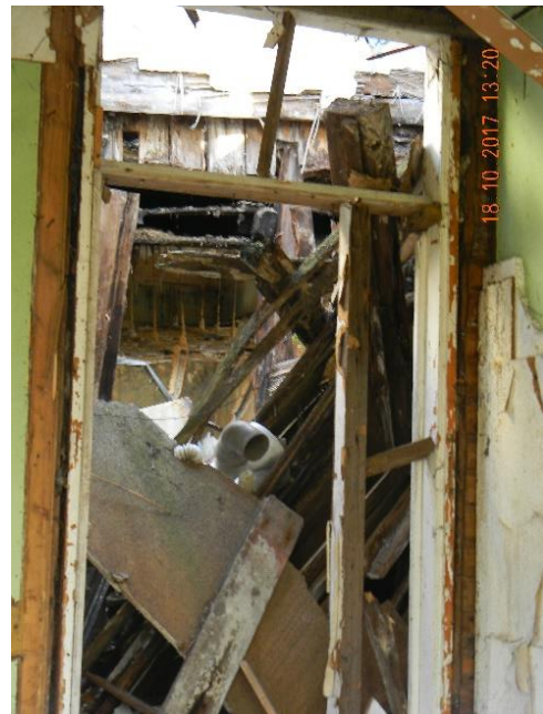
Figure 1. Ruined building at Kościuszki 29 Street: A- veranda, current state, B- collapsed ceiling inside.
