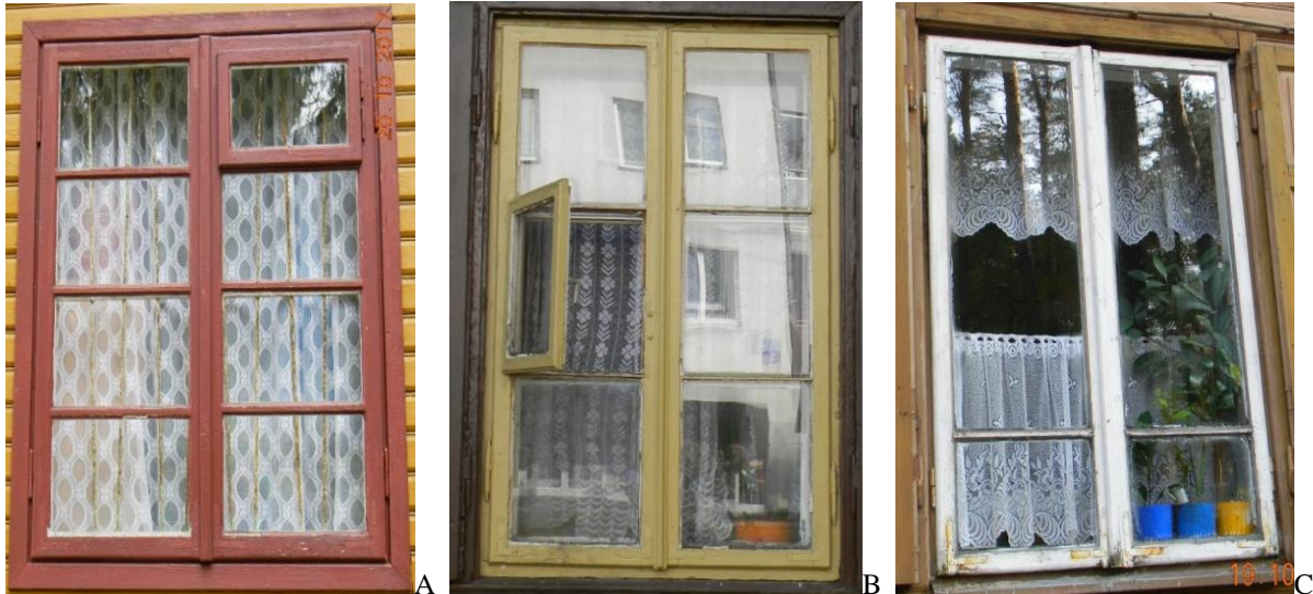
Figure 8. Windows with "vents" (small casement parts opening independently): A- Jana Pawła 13 (No.13), B- Samorządowa 8 (No.66) and a window with mullions placed in its lower part: C- Czarnieckiego 6 (No.6)
