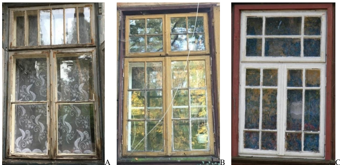
Figure 4. Windows with mullions above and below the transom A- Willowa 6 (No.77), B- Świerkowa 16 (No.73), C- Mała 5 (No.37)
