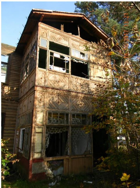
Figure 1. Ruined building at Kościuszki 29 Street: A- veranda, current state, B- collapsed ceiling inside.
