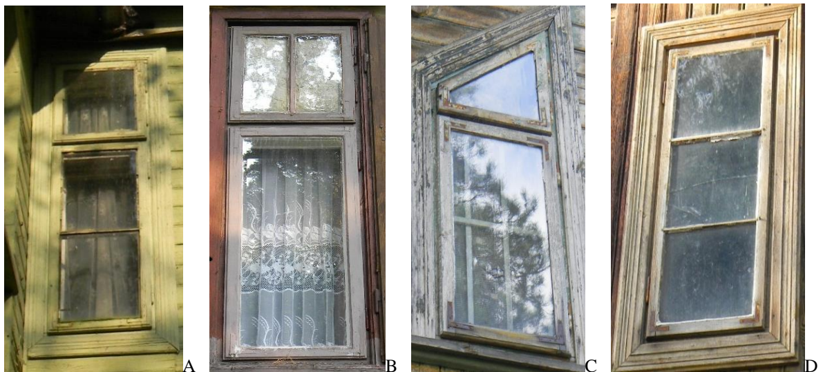
Figure 9. Single-unit windows with transom: A- Mała 3 (No.38), B- Piaskowa (No.57), C- Poniatowskiego 11 (No.63) and a single-unit window: D- Jeremy 5 (No.14).
