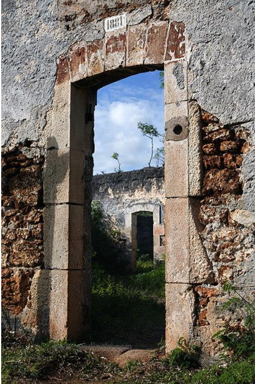
Photo 4. Prison gate in Ouro, Isle of Pines
