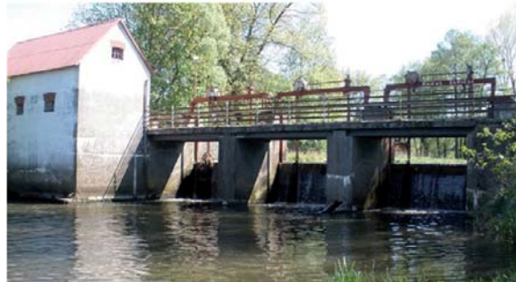
Small hydropower plant in Kamion village (km 37.8).
