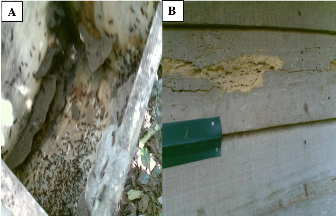
Figure 2. Honeybee's Hive (A) and food canteen stall (B) attacked by carpenter ants and powder post beetles, respectively.
