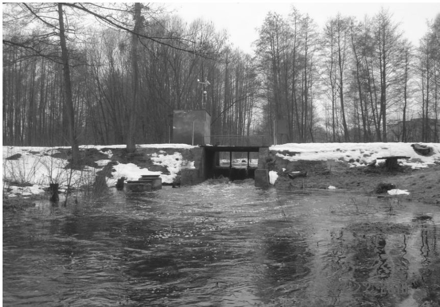
FIGURE 3. View of the stream gauging station at Czarna (photo is looking upstream and was taken during snowmelt period at discharge, which is close to the 2-year flood)
