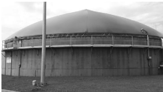
Figure 1. Large-scale semi-buried digester located in north-eastern Poland
