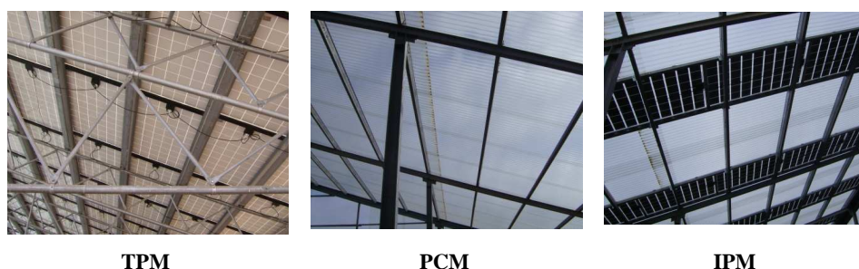
Fig. 1. Details of greenhouse cover material: (TPM) traditional photovoltaic modules; (PCM) polycarbonate modules; (IPM) innovative photovoltaic and polycarbonate modules
