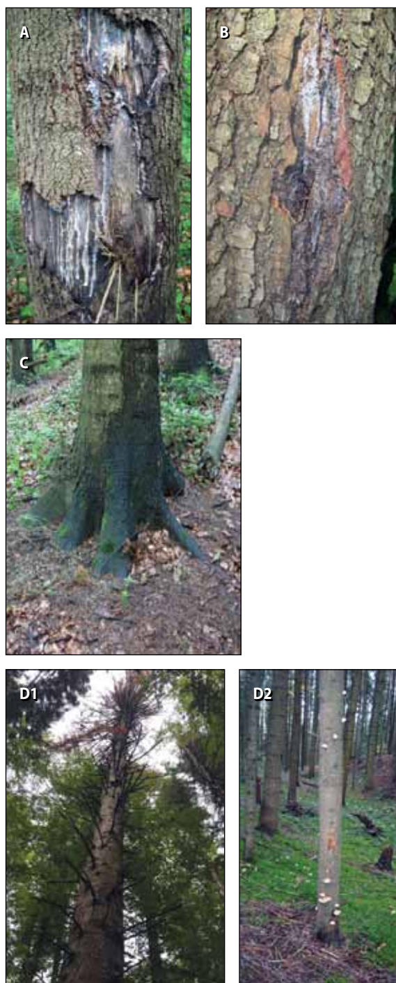
Figure 1. Macro-signs of bacterial wetwood disease in Abies alba : A – cracks and exudate on rhytidome; B – ulcer formed with exposed secondary phloem and wound meristem (callus); C – wet base of the trunk; D1 – dieback of epicormic shoots; D2 – settlement of secondary pathogens
