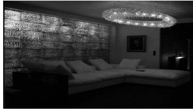
Fig. 5. Wall made of the translucent concrete Litracon [21]
