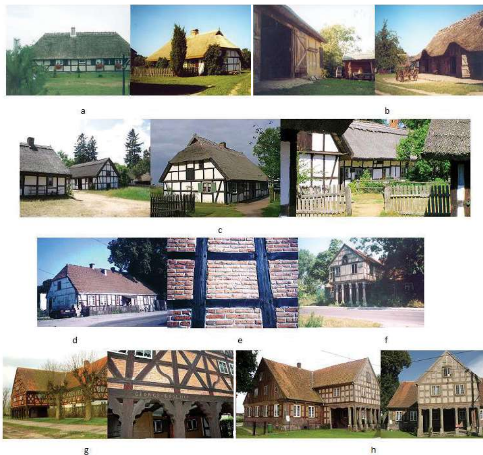
FIGURE 1. Selected examples of the ancient skeleton construction: a—Cassubian hut from 1802 rebuilt in 1984, Karwieńskie Błota; b—Cassubian hut, barn and cowshed in an antique rich farmer's farmstead, Nadole; c—farmstead buildings, Kluki; d—dwelling house, Smolno; e—a detail of a post-and-beam wall filled with ceramic brick in a farm building from the end of the 19 th century, Darżlubie; f—canopy house from the beginning of the 19 th century, designed by a Gdańsk architect Piotr Loewen, Żuławki, Warmia; g—canopy house from 1720, Trutnowy; h—canopy house from 1840, Nowa Kościelnica (photo by Mirosława Górecka)
