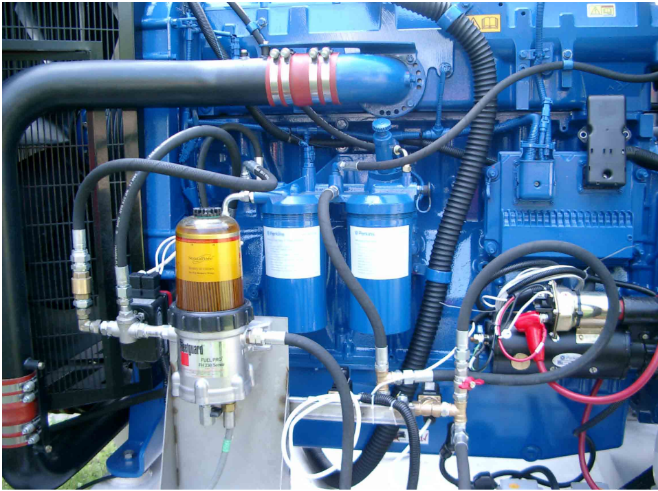
Phot. 2. Engine Perkins 2806A-E18TAG2 with a special, heated rape oil filter. View of a part of supply system.
