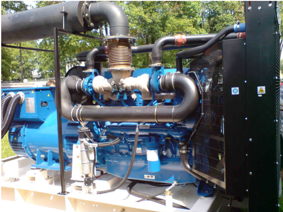
Phot. 1. Overall view of the generating set with the examined engine Perkins 2806A-E18TAG2
