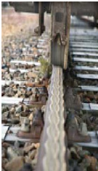
Fig. 1. Presence of residues of sand on rails
