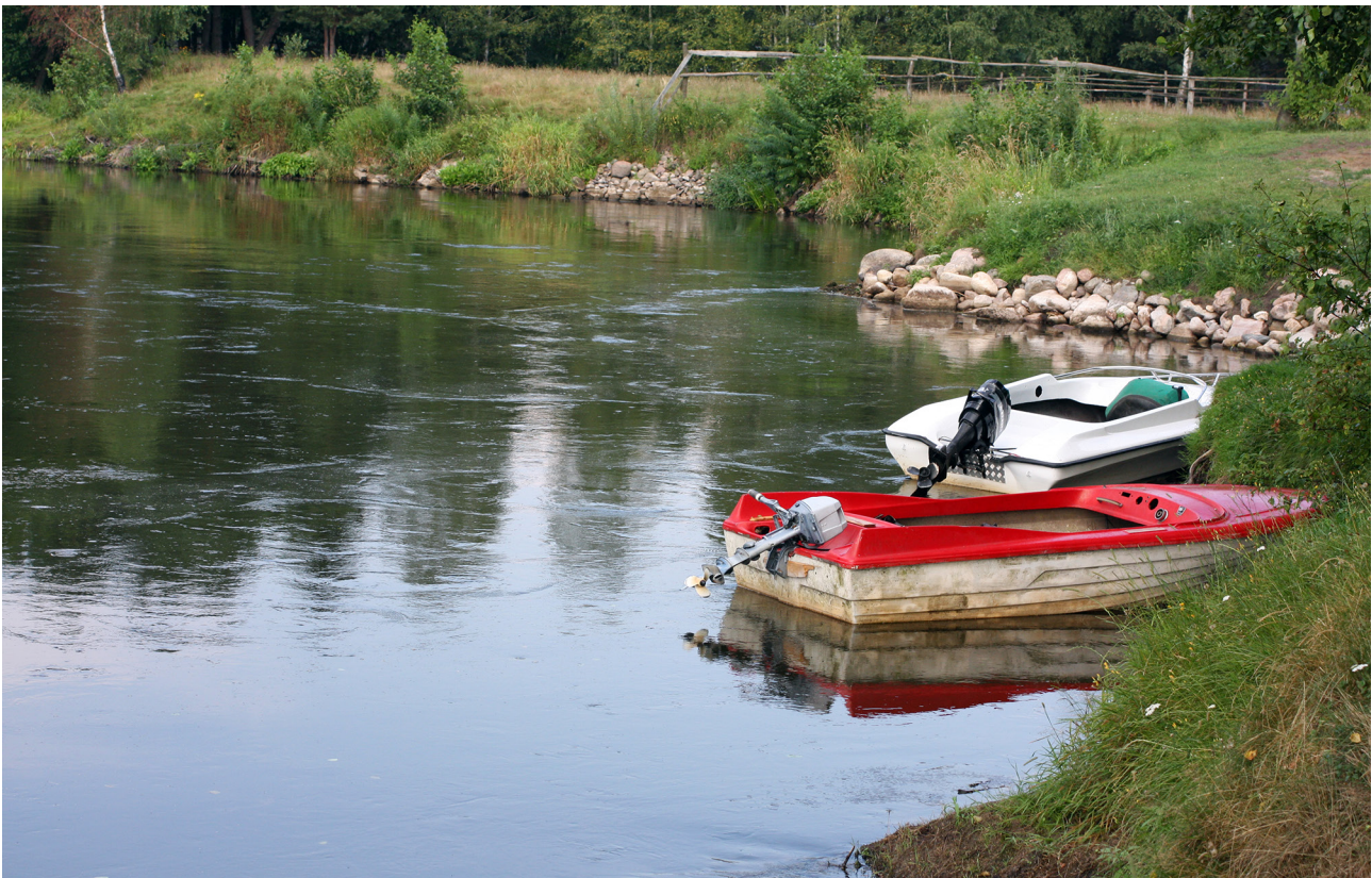
Fig. 4. Riverbank revetments made up of armour rock in the vicinity of Ciecioro village (July 2014). Photo: A. KAMOŃKI
