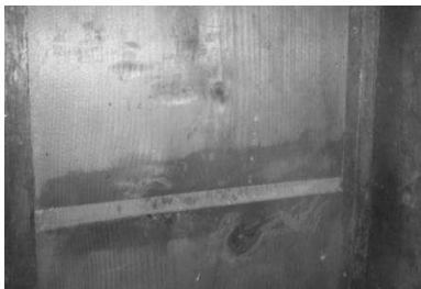
Figure 27. Groove joint on the left side
