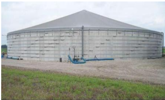
Fig. 4. Stainless steel manure pit
