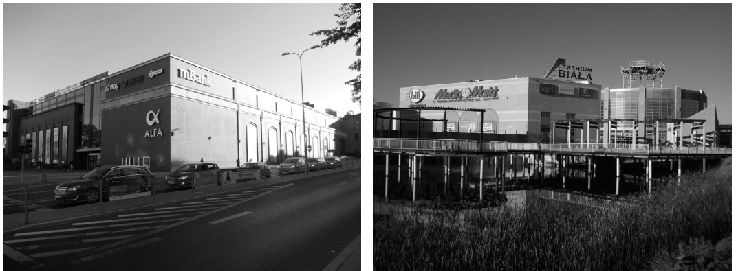
Figure 1 and 2. New commercial function allowed to create attractive popular places of shopping and in some aspect of social interactions and functional activation of surroundings. Alfa Shopping Center and Biala Shopping Centre in Bialystok
